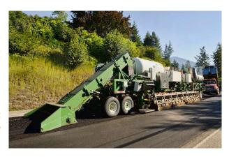
HIP is used to treat surface cracking, raveling, potholes, and rutting. It can also address problems such as bumps, swells and depressions that affect ride quality.
