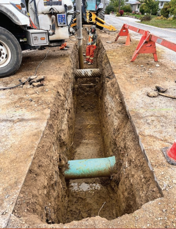
▲ Scott Street Storm Line Installation
