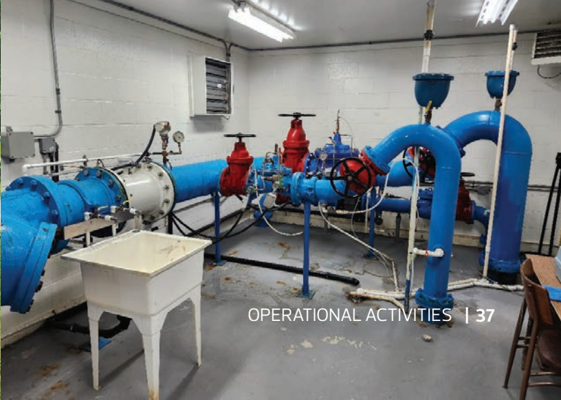
▼ Flow Meter installed at Crawford Hill Reservoir
