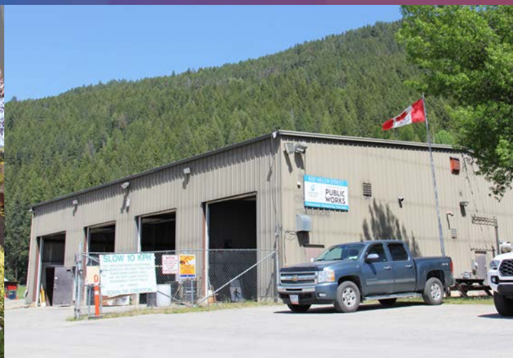
Public Works Building ▼
