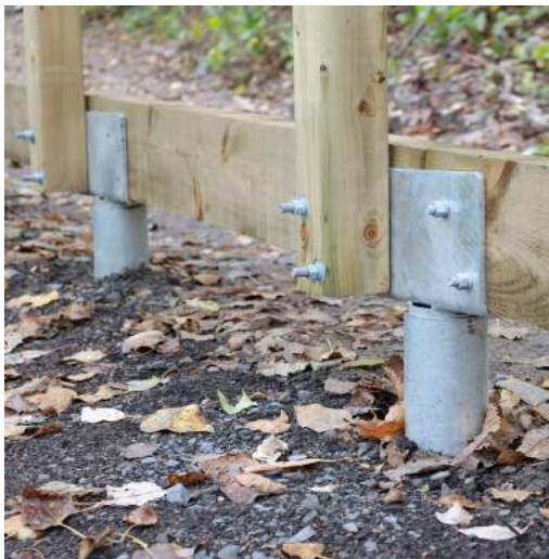
..... Left: Helical pile foundation .....
