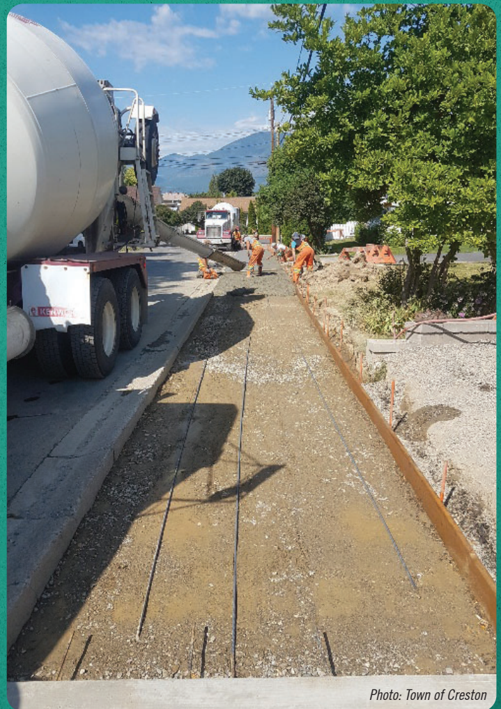
Installation of new sidewalk on Cedar Street
