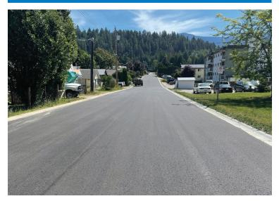
Hurl Street between 16th Avenue N and 19th Avenue N has been rebuilt. The project started last fall and was recently completed. The street road base was significantly deteriorated, requiring a full rebuild of the road base and repaving. This was completed, as well as curb and gutter replacement on south side of the street. The water infrastructure was identified for upgrading, which was what prioritized this project over other streets.
