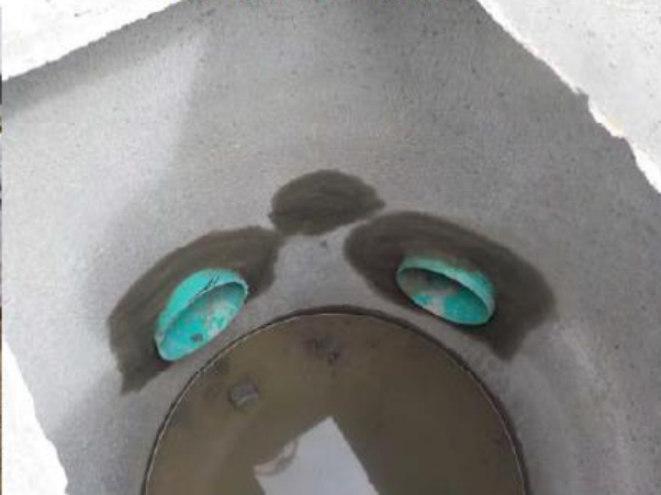
Grout CB 1007 Inside
