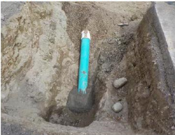
100+180 CB Lead tie in & Grout
