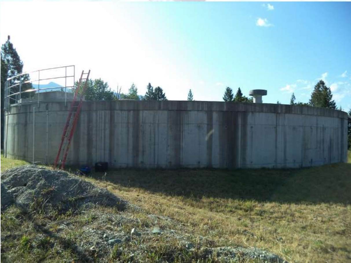
Crawford Hill Reservoir
