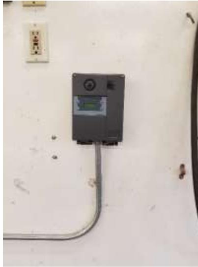
**FIGURE 4: EXHAUST DETECTION SYSTEM**
